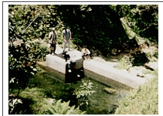
Figure 10-4 A concrete weir can be used to form a small reservoir (Nepal).
