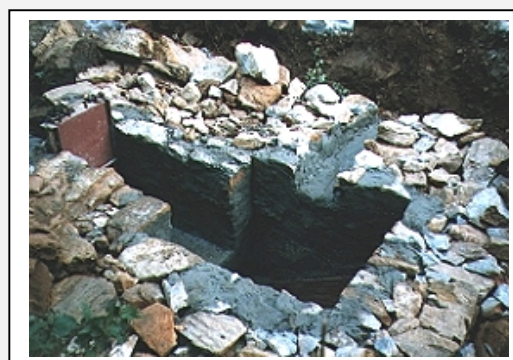
Figure 10-16 The flow of water into the forebay is controlled by a sluice gate. An overflow is cut into the wall on the downhill side so that excess water is returned to the stream without undermining the masonry. A flushing pipe, sealed with a wooden bung has been incorporated at the lowest part of the tank.
