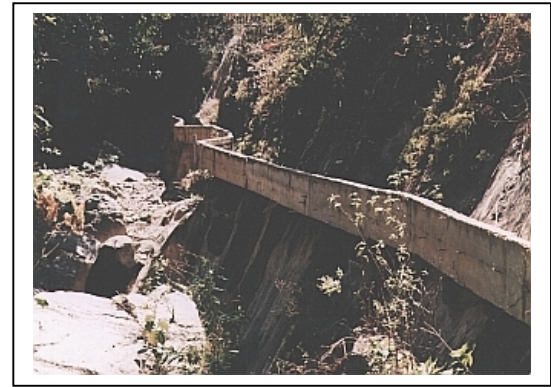
Figure 10-6 Canal installed in a difficult location supplying a small hydro scheme for local electrification (Peru)
