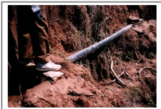
Figure 10-7 A length of pipe can be used to bridge a difficult gully with a small canal. The pipe is secured with rocks on either side.
