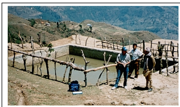
Figure 10-17 A small reservoir provides low-cost energy storage which can be useful during the dry season. (Sankhuwa Sava, Eastern Nepal)
