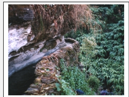
Figure 10-9 and Figure 10-10 show a raised canal that runs on a narrow ledge underneath a vertical rock face. The canal has a masonry lining and is supported by a high stone wall underneath.
