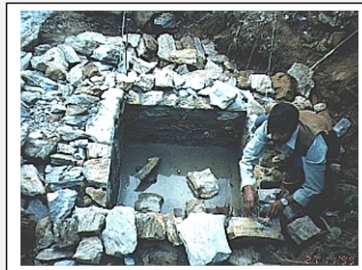
Figure 10-15 Construction of stone forebay (Kushadevi, Nepal)
