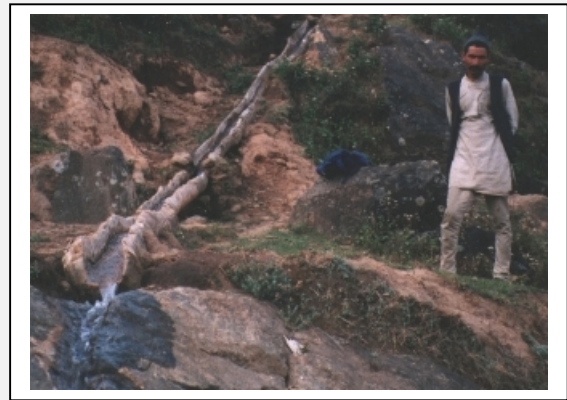
Figure 10-8 A wooden aqueduct can be used to transport water in the canal across uneven ground
