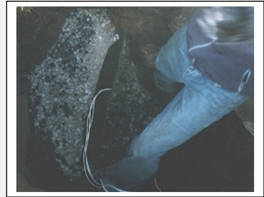
Figure 9-3 Installation of a copper-plate earth electrode, Multiple earth cables have been soldered in place to reduce the resistance and increase the reliability. (Nepal)
