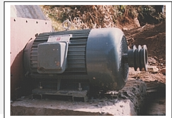
Figure 9-4 3-Phase Induction Motor (7.5 kW) with double-ended shaft, used as a generator. (Nepal)
