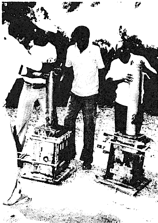
The construction of chimney segments.
