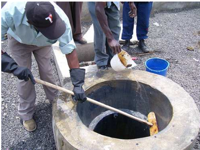
Figure 8. Maintenance of biogas settler at Naivasha bus park in Kenya: Cleaning of the manhole of the biogas settler from old clay to prepare for re-sealing (source: C. Rieck, 2009) 10 .
