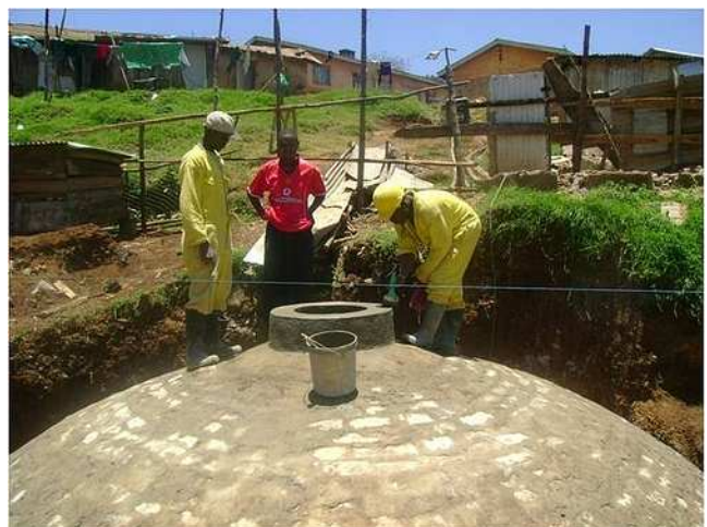
Figure 1. Construction of biogas digester at Meru prison, in Meru, Kenya – type: biogas settler, fixed dome (source: S. Blume, 2009)
