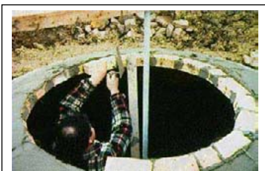
Figure 3: Fixed-dome plant in Tunisia. The final layers of the masonry structure are being fixed.
