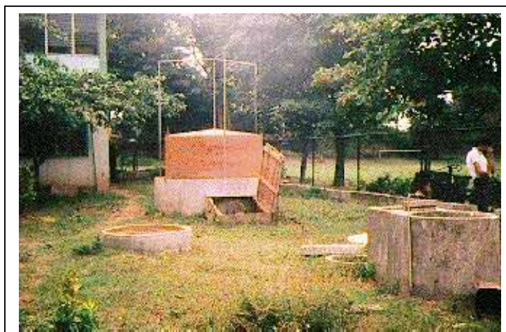
Figure 18: Biogas plant with separate gasholder in Nicaragua
