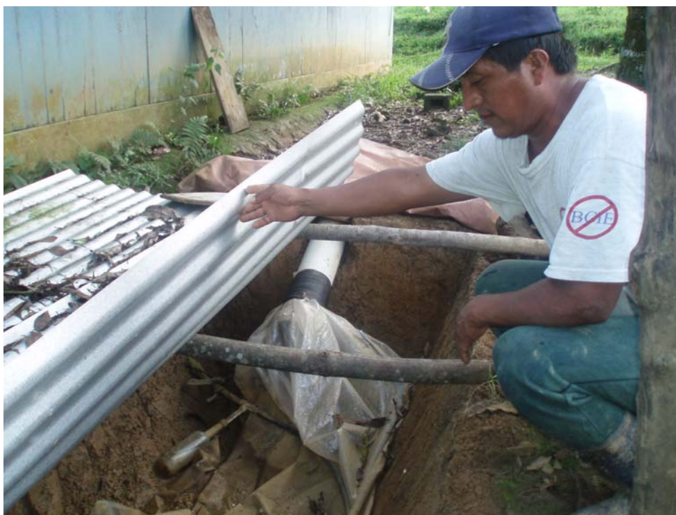
Figure 18. A failed biodigester in Chiapas pushes a negative stereotype of the technology for the local community.
