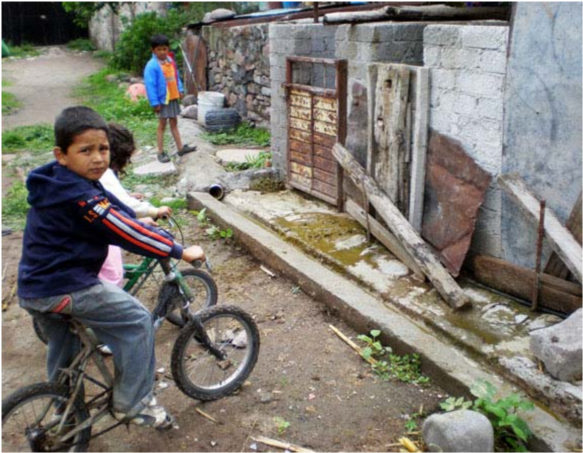
Figure 36. The same site as in figure 35 is shown here after the biodigester installation. Waste is contained and transported to the biodigester through collection canals.
