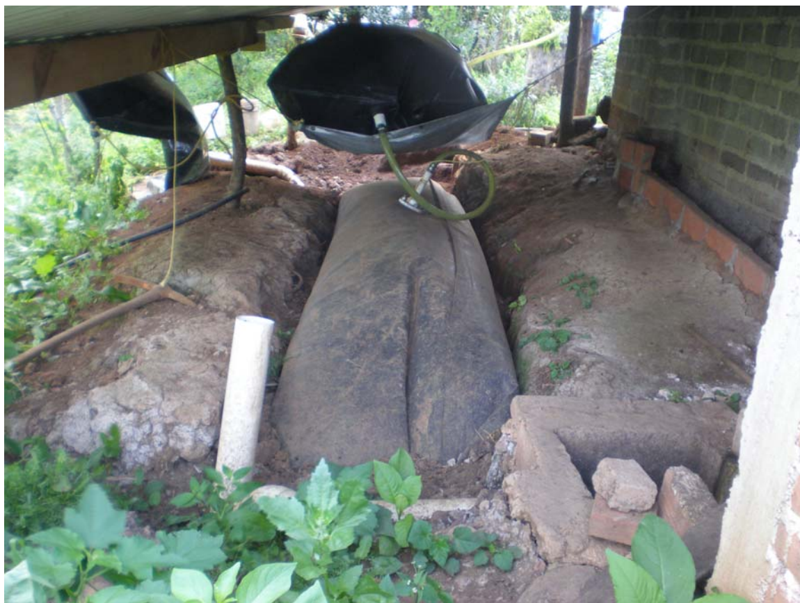
Figure 27. The same digester as in Figure 25 and 26 is shown here after it was untwisted, with the waste entrance and exit pipes at the site modified to accommodate the corner mounted exit and entrances of the biodigester.
