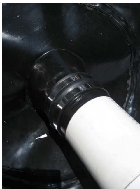
Figure 24. A closer look at the inlet and outlet design for liquids shows the double four-inch hose clamp sealing the PVC pipe to the biodigester body. This PVC tube continues into the biodigester about 40 cm.
