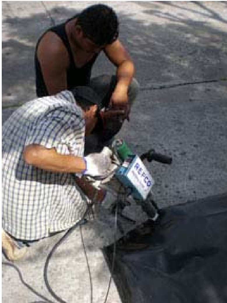
Figure 28. The HDPP extrusion welding gun can be seen here sealing the HDPP Eviroliner in San Luis Potosi, Mexico.
