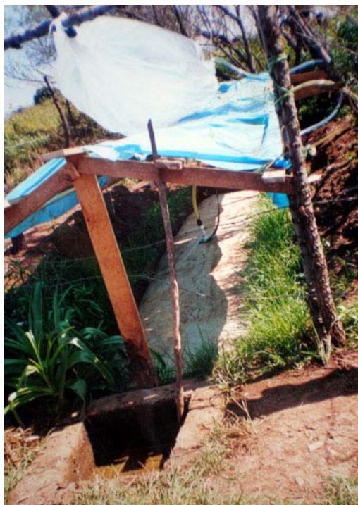
Figure 10. An early plastic biodigester installed by a course in Colombia attended by Ms. Nambo in 1997.
