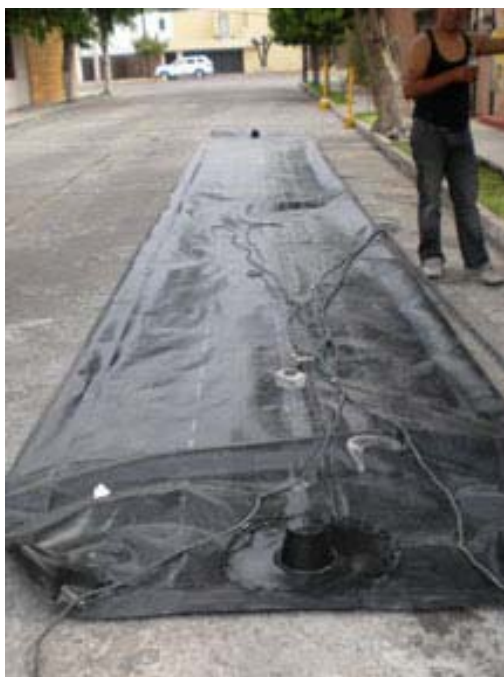
Figure 29. The first improved biodigester made from HDPP Enviroliner. In the foreground a new PVC adaptor sleeve can access port can be seen. This is a 10 m improved biodigester.
