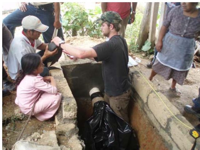
Figure 13. The mouth of the tubular plastic is folded around entrance and exit tubes and secured initially with tape before it is wrapped with tire inner tube. This is a system in San Jose Zapotal, Chiapas.
