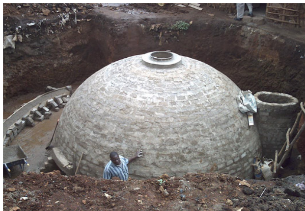
Figure 5. A fixed dome biodigester under construction at the Mukuru BioCentre in Kenya. The high technical skill needed to construct these systems is apparent here (photo: Dyfed Aubrey).
