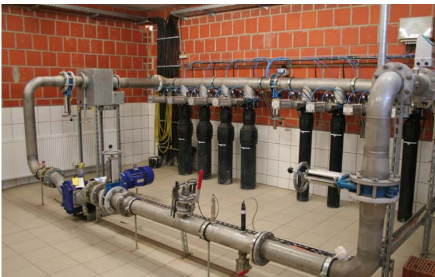
Fig. 3: Central pumping station of a biogas plant in Lelbach with online sensors (front)
