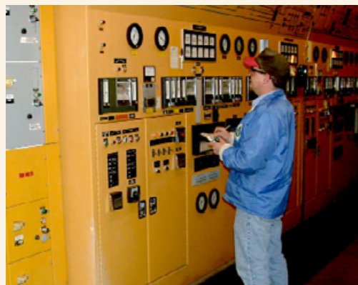
Digester controls at a wastewater treatment plant
