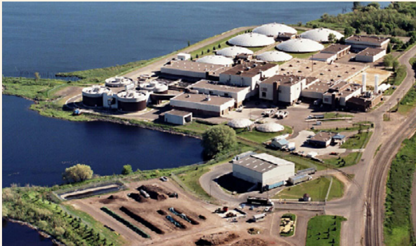
Western Lake Superior Sanitary District wastewater treatment plant in Duluth, MN
