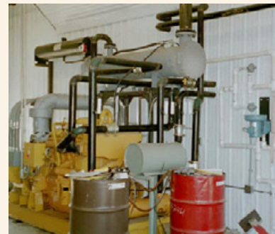
Digester engine with heat recovery system
