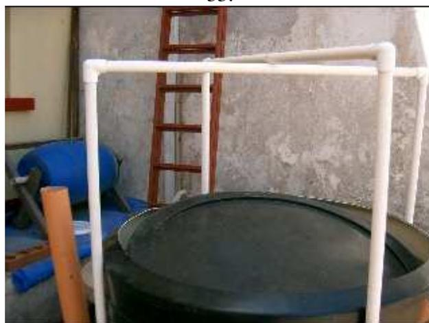
To prevent the gas holder (the smaller tank) from rising too high, a structure is attached to the outer tank as shown in photo 33. Three lengths of 1" PVC pipe are connected together with 90° elbows to form inverted 'U' shapes (140cm → 129cm → 140cm.) This is built twice. The two structures are connected over the biogas digester in an 'X' formation.
