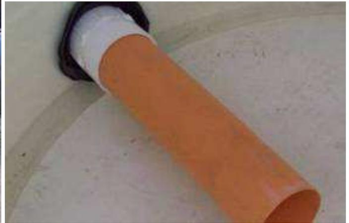
As shown in photo 23 the inlet should be extended on the inside of the tank.
