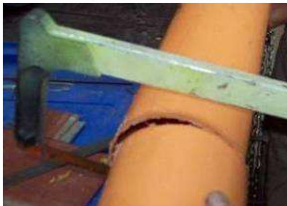
Mark the 4" PVC pipe to size and cut it with a hacksaw. The lengths are shown in photo 17.
