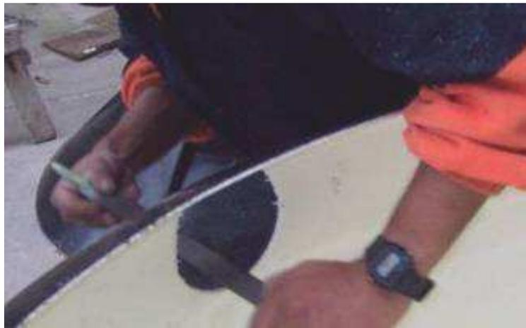
Holes in the tank for the inlet and outlet are made using a jigsaw:
