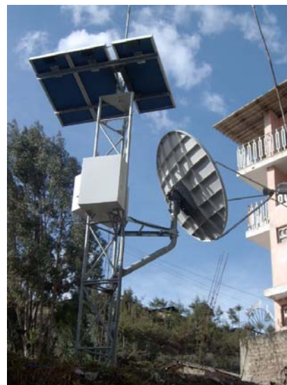
Figure 3: The La Encanada infocentre, Peru. It has solar panels to generate electricity and a satellite for connectivity.
