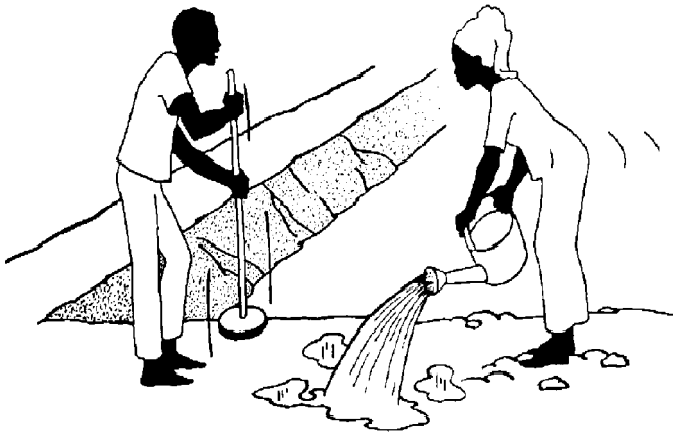
Figure 32: Compacting the dike (Viveen et al., 1985).
