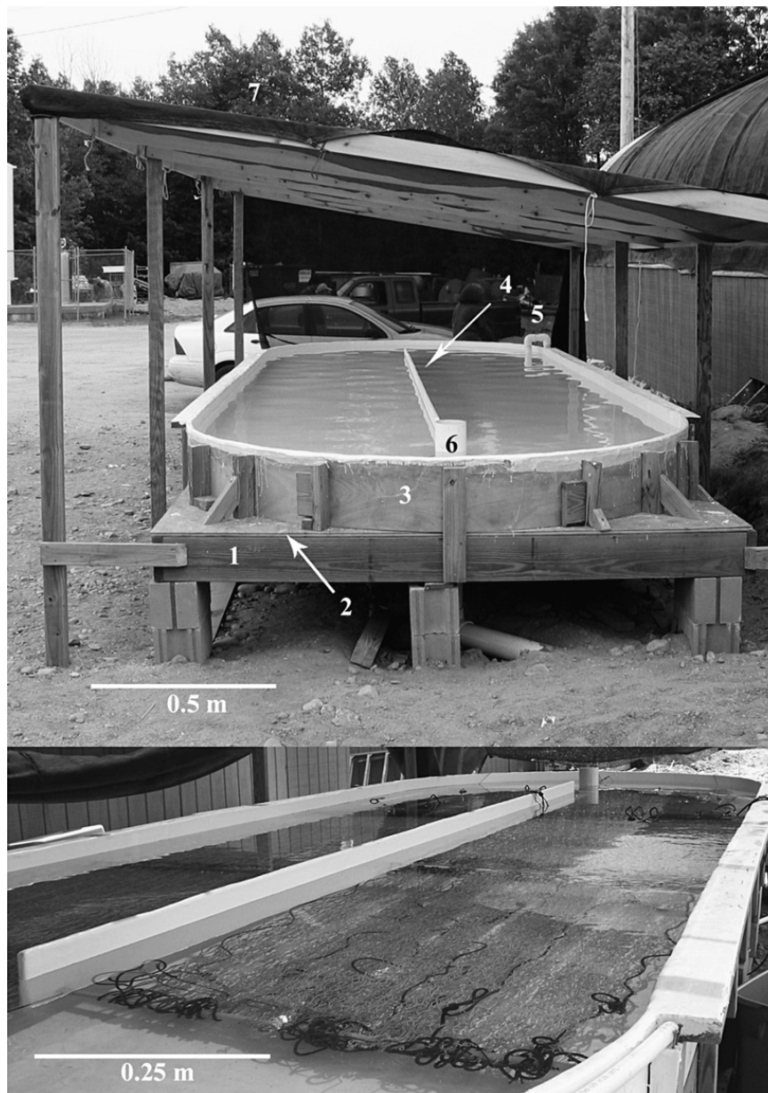
Fig. 1. Image showing the layout and construction of the raceway (top) and method of suspending the nets in the raceway using PVC pipes (bottom). 1) Deck; 2) sheathing; 3) curved radius; 4) center divider; 5) make-up inflow; 6) standpipe; 7) shading.
