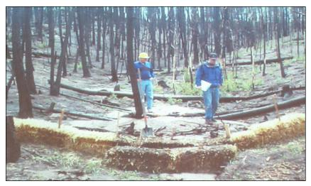
Contour felling of small diameter trees on slopes, and tree trunks and straw bales in swales are inexpensive and effective erosion controls.
