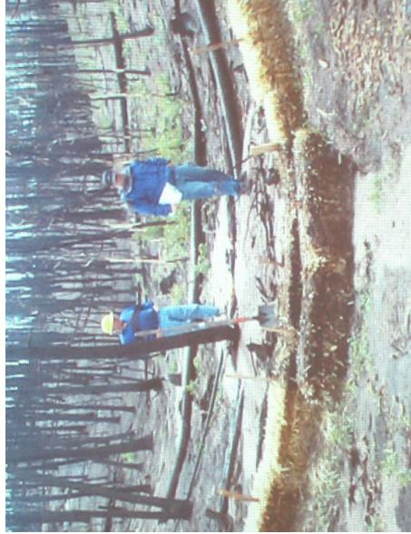
**Contour felling of small diameter trees on slopes, and tree trunks and straw bales in swales are inexpensive and effective erosion controls.**
