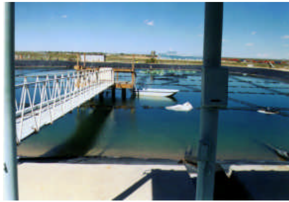
Figure 6: Picture of Solar Gradient Ponds at El Paso, Texas. Note the netting on surface.
