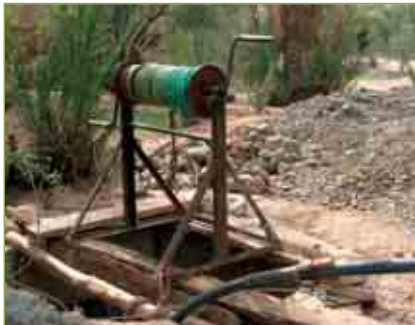
Building a well, Morocco
