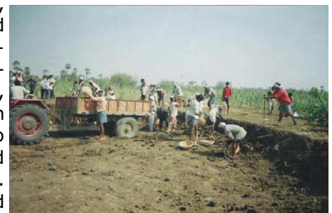
Tank desiltation - Local people at work
