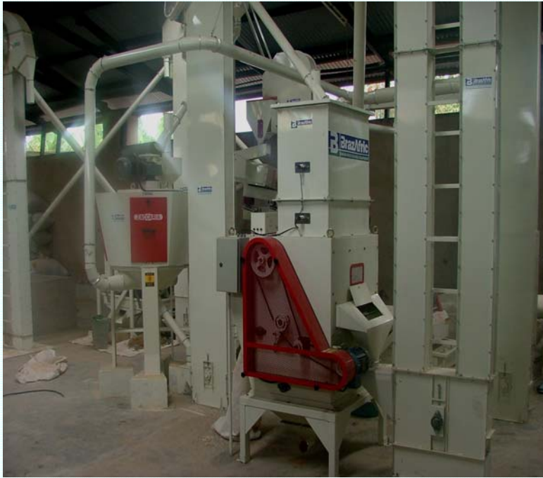
A medium-scale rice processing plant in Kasana, Luwero district, installed by Savannah Commodities, an APEP-SAF client.
