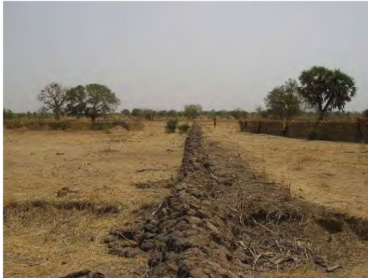
Gabion, province de la Tapoa, Burkina Faso
