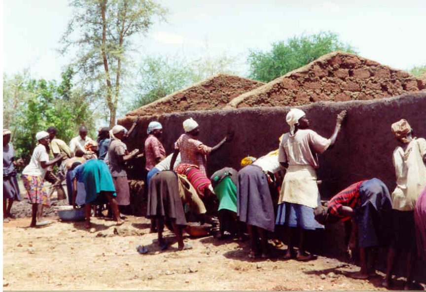
Figure 1 – Plastering house with mud mixed with ‘sour water’
