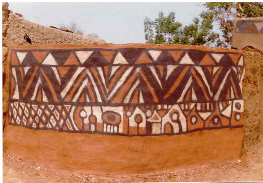
Figure 13 – Traditional house in Kandiga with colored plaster made with ‘sour water’
