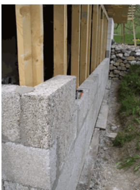
Concrete block made with hemp in France
