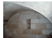
Hemp interior thermal insulation blocks
