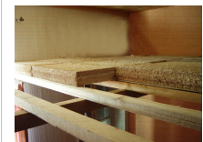
Hemp acoustic ceiling insulation
