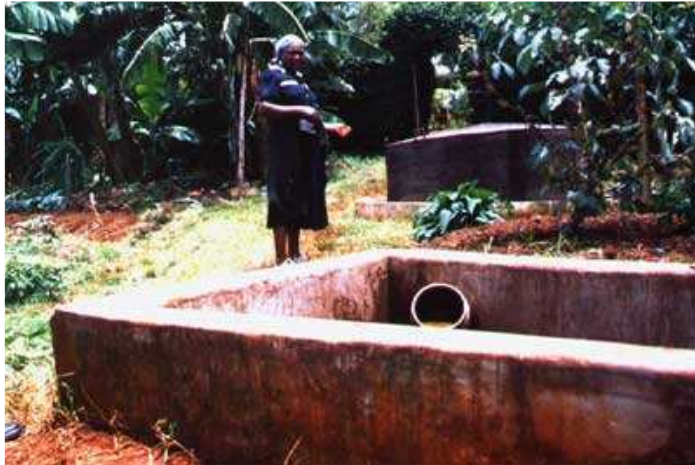
Figure12. Mrs Okido shows her biogas unit that produces methane for her cooking and lighting and slurry for fertilizing crops
