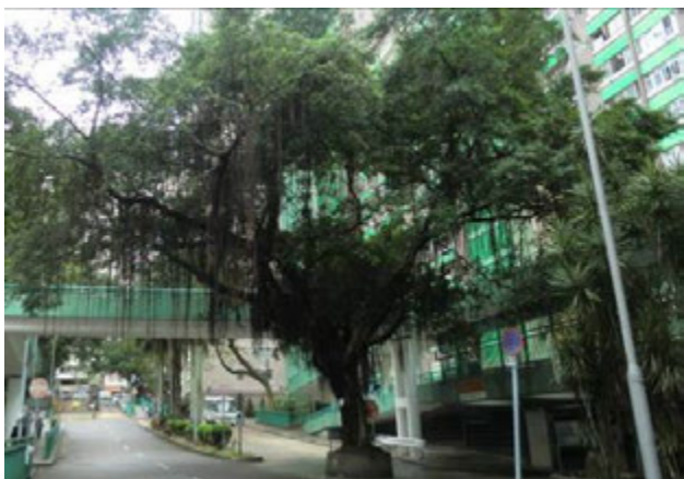
Photo no. 1 - Overview
