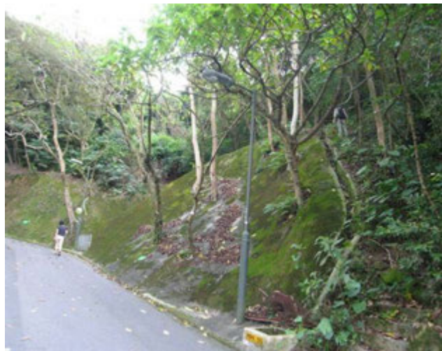
Photo no.1 - Site condition
