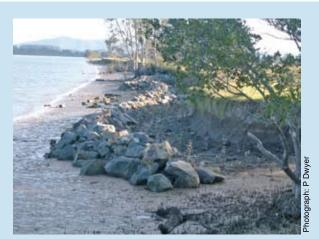
Figure 21. Rock fillet method at Hastings River, mid north coast NSW.
