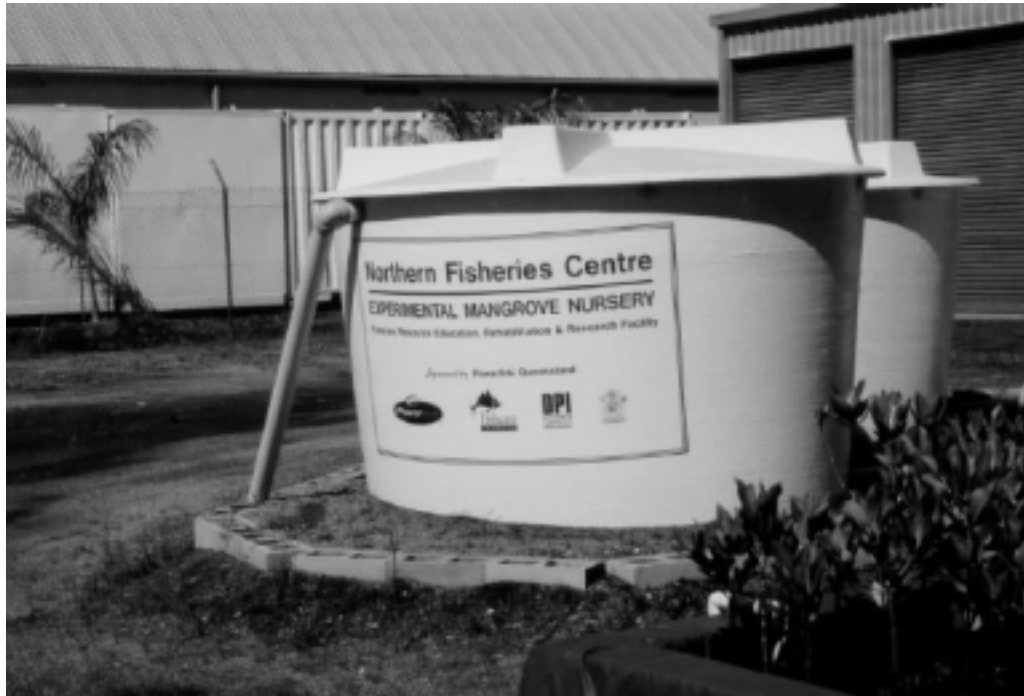
Plate 3. Saltwater Reservoir tanks (5000 litre), Cairns QFS nursery
