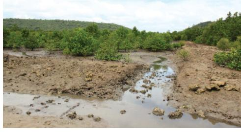
Strategic breaching involves intentionally making holes in dike walls, with the intention of creating, over time, a natural meandering drainage channel. These breaches are narrow at the landward side, widening as the approach the coast. The resultant tidal creeks should meander, i.e. do not create strategic breaches in a straight line. (see Fig 8.7)
