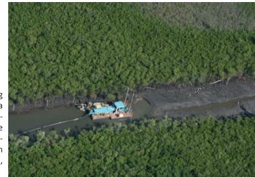
Fig 8.4: Floating dredge restoring a tidal creek to improve tidal exchange which is causing dieoff of mangroves in Tampa Bay, Florida, USA, (Lewis).
