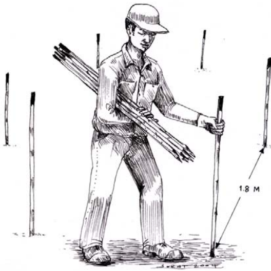
1. Stake out the site.
