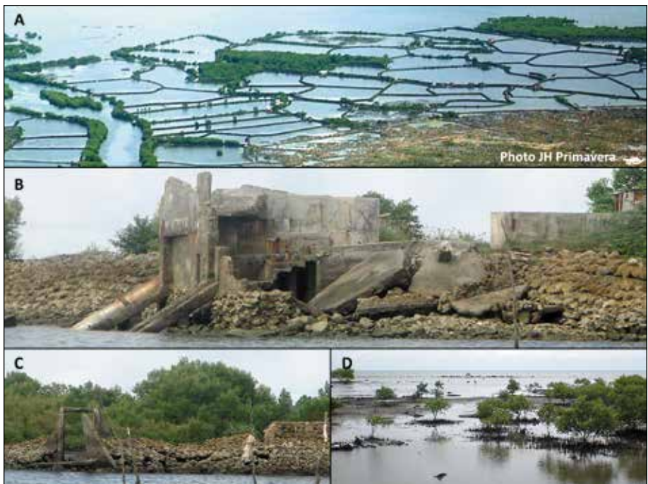
FIG. 23. Increasing typhoon frequency and severity cause progressively greater damage to coastal fish ponds (A, D). A mangrove greenbelt (C) is the most cost-effective alternative to bigger budgets to repair dikes and gates (B) such as in Dumangas, Iloilo.
