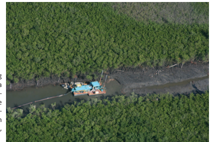
Fig 8.4: Floating dredge restoring a tidal creek to improve tidal exchange which is causing die-off of mangroves in Tampa Bay, Florida, USA, (Lewis).
