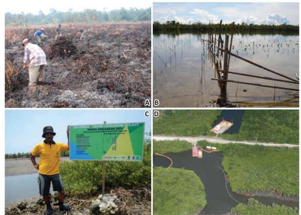
Fig 8.2: Some site preparation measures include: clearing Acrostichum and levelling mud lobster mounds (A), fencing (B), posting signage (C) and placement of turbidity control screens (D).
