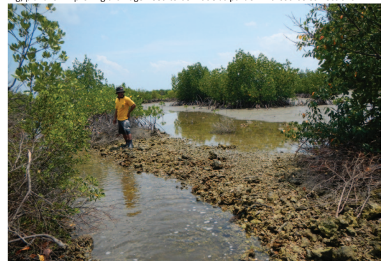
Fig 5.18 Hydrological Disturbance - Although this dike wall was levelled during initial rehabilitation, it is still high enough to block drainage of the pond (background) into the tidal creek (foreground). After identifying continued hydrological disturbance during monitoring, plans for improving drainage need to be made as part of mid-course corrections.
