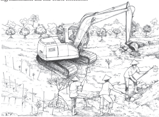
Fig 8.1: A choice needs to be made between use machinery and employment of community labor with hand tools. At smaller scales (<50 ha) community labor may be sufficient, while larger scales almost certainly require heavy equipment.
