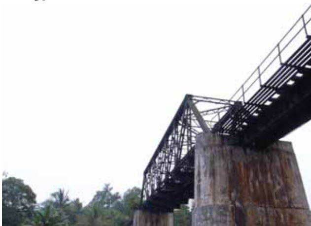
Cast iron railway bridge across the Sungei Ulu Pandan
