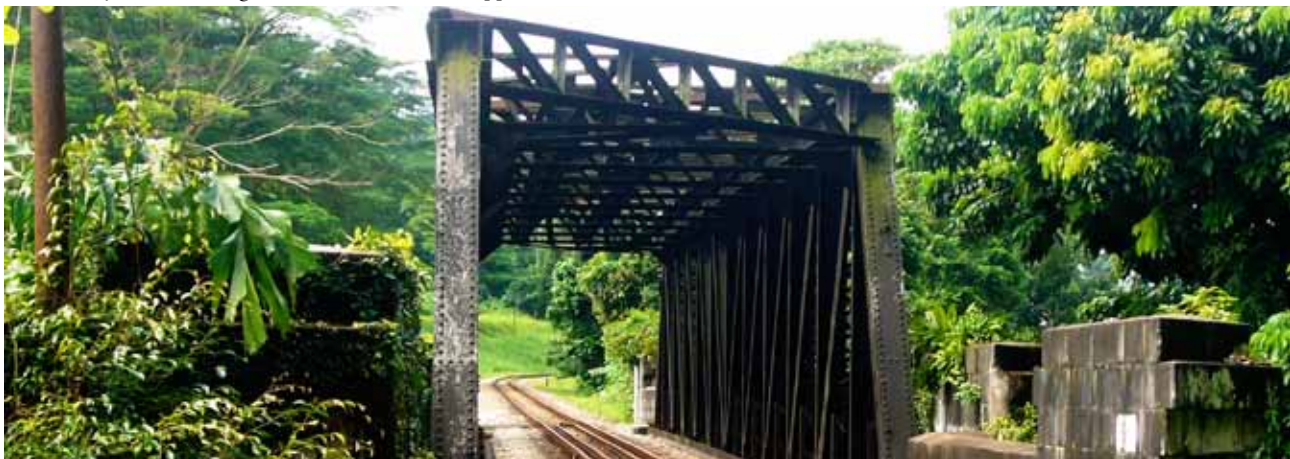
Cast iron bridge over Upper Bukit Timah Road
