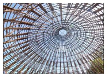
The dome was built out of bamboo poles, then covered with a thatched roof. Vietnamese timber bamboo, bambusa stenostachya, was the first bamboo pole to be certified for the International Building Codes. These poles are very hard wood and are 3-4" diameter with thick walls.
