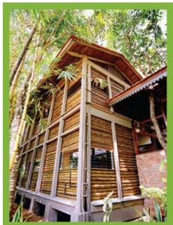
We were able to reduce the use of 70 to 80% cement and steel, by the use of bamboo, if we are to compare with a building of same design built with conventional materials.
