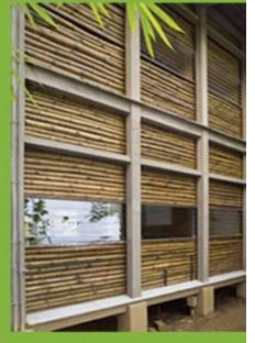
Probably the first and largest of its kind in India, Inspirations' office is built almost entirely with engineered bamboo – be it the floor and roof slabs and the walls The office covering an area of about 2750sqaure feet was completed in Dec. 2002. It is noteworthy that almost 25% of the bamboo used in the building was obtained from the neighboring bamboo plantation. All the bamboo used for this building was treated with preservative treatment to meet functional requirement.
