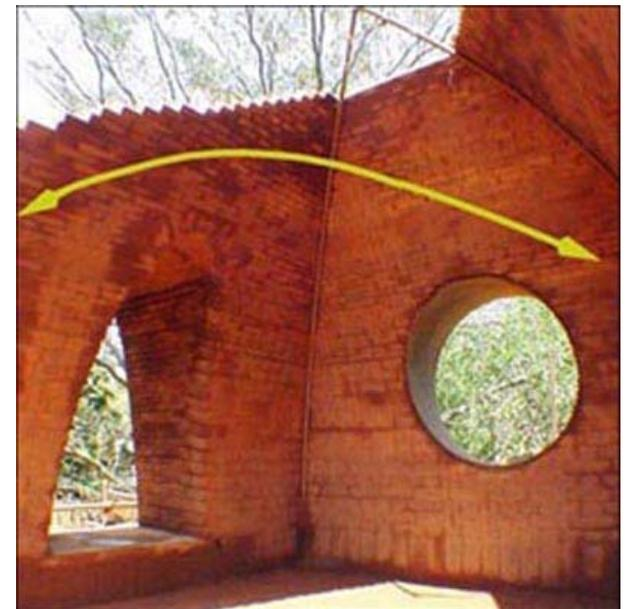
*Load transfer in the shape of a catenary in an equilateral vault with a half dome*
