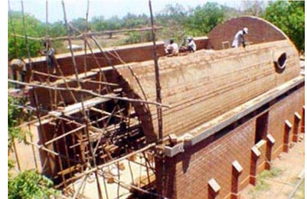
*Building a semicircular vault of 6m span*
