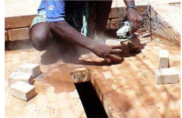
3. Grind a block to adjust its length
