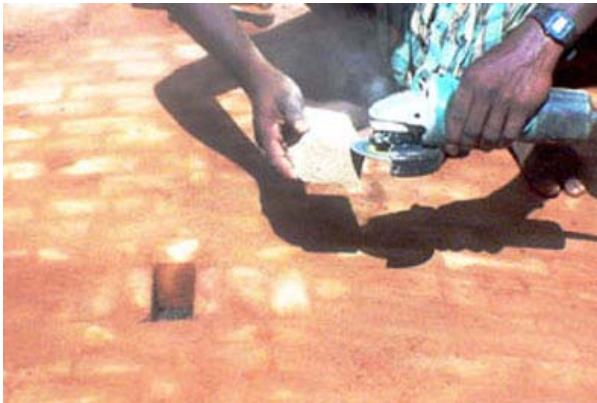
8. Grind the keystone to adjust its thickness
