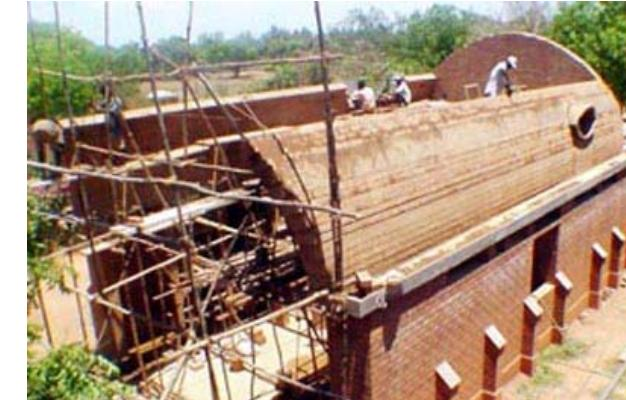
*Building a semicircular vault of 6m span*
