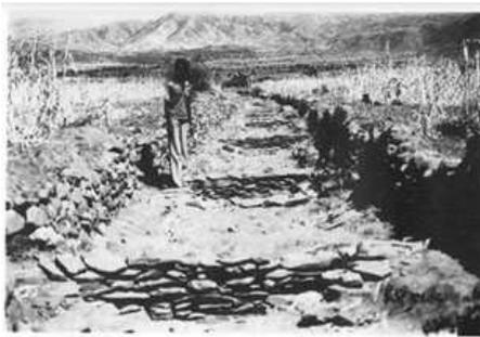
Plate 5.35 Flood diversion structures, Tigré, Ethiopia, taken at point A on Figure 5.14 (J. Bennett, Arden Press Agency)
