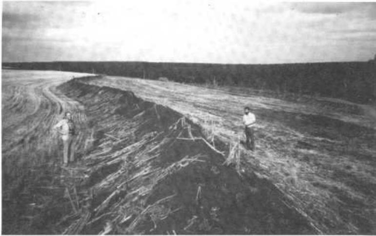
Plate 4.10 Murundum terrace in Brazil, intended to hold all surface run-off, even during heavy storms (T.F. Shaxson)
