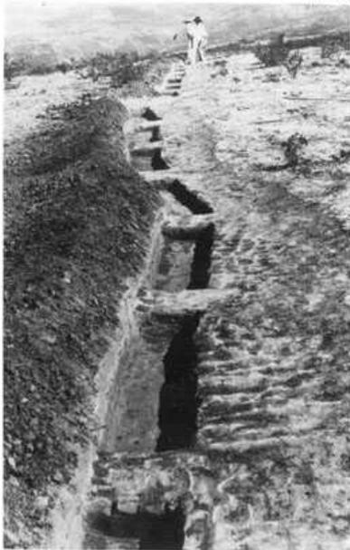
Plate 4.16 Hillside ditch with lock and spill drain (USDA)
