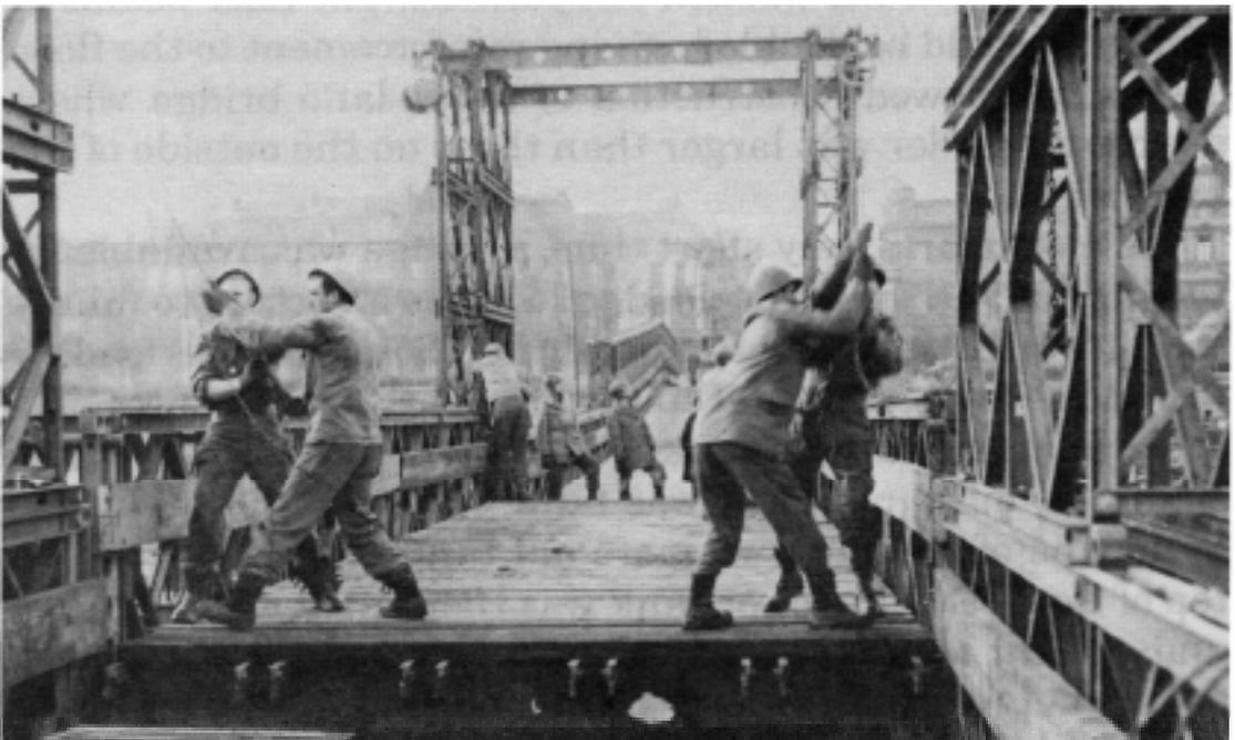
*Engineers lift the bascule span of a class 70 Bailey bridge.
