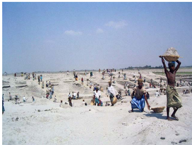
Figure 8: The whole community work together to make a large raised platform for the cluster village. Photo: Practical Action Bangladesh.
