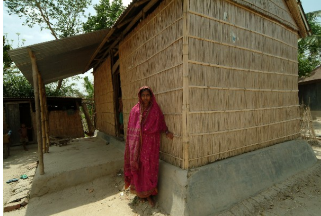
Figure 3: Julekha Begum is the owner of this house in Yasin Mirdhar Dangi, Faridpur. Photo: Practical Action Bangladesh.
