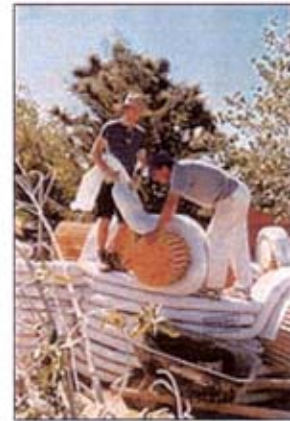
Bags filled with earth are moulded to the shape of the building.
