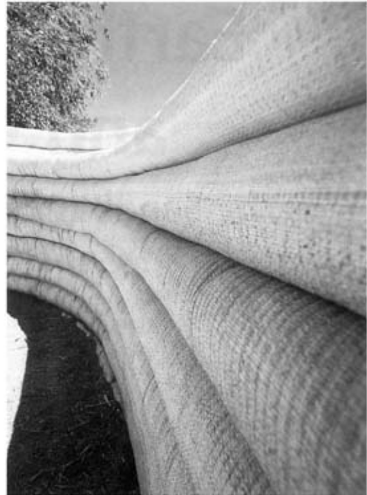
Wall of Superadobe construction—earth-filled sandbags and barbed wire. Coils/courses can be filled by hand or by pump at speeds of 10 to 15 feet per minute, depending on bag width.
