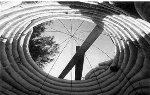
Double-curvature compression shell, or dome, of Superadobe construction showing rebar guides for the dome shape (removed later) and a simple plank scaffold. Gravity is the generator of the form.
