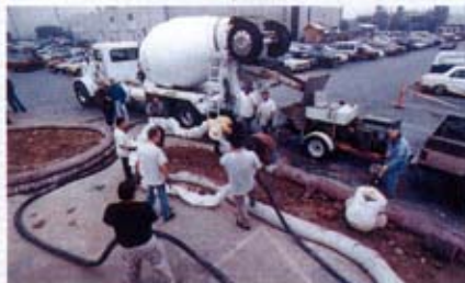
Superadobe/superblock coils under construction, demonstrating pumping method.
