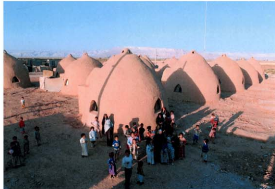
Phase II: After a prototype domed shelter was completed at the Tehran Building Research Center, fourteen Sandbag Shelters (domes only) were constructed by the refugees themselves in 6-11 days, with UNDP supervision. The refugees immediately moved into the shelters, and some upgrading was completed soon afterwards (plaster finishes, windows and doors).
