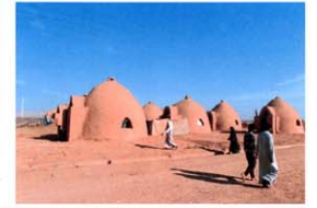
Phase II: After a prototype domed shelter was completed at the Tehran Building Research Center, fourteen Sandbag Shelters (domes only) were constructed by the refugees themselves in 6-11 days, with UNDP supervision. The refugees immediately moved into the shelters, and some upgrading was completed soon afterwards (plaster finishes, windows and doors).
