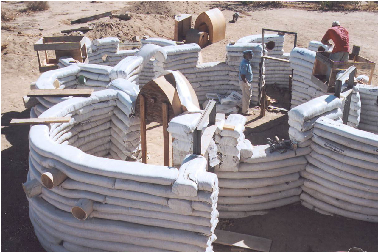
Demonstration of the construction of domes with multiple niches and rooms using the “superadobe” method that meets United Nations standards.
