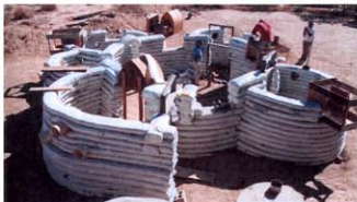
Upgraded Shelter Dome with Apses under construction
