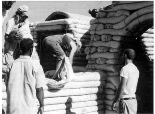
Trainee builders work with hand-filled Superadobe. Long sandbags are filled with earth from the site and tamped in place on the wall. Between courses are set two strands of four-point barbed wire.
