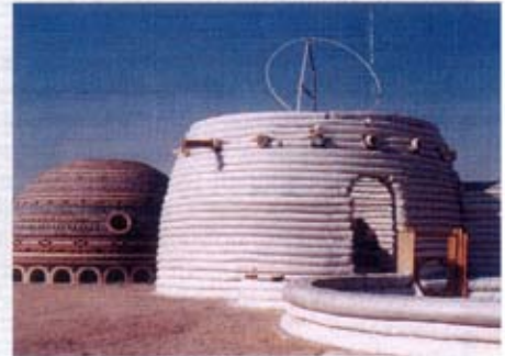
Hesperia Museum and Nature Center utilizes 91 percent in-situ materials to construct stabilized superadobe/superblock coils, with both pumping and manual systems.
