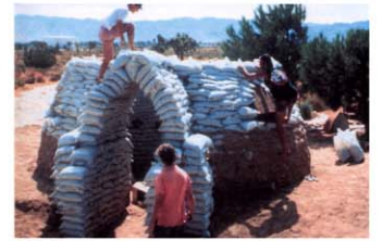
Original tested prototype dome under construction, 1992.
