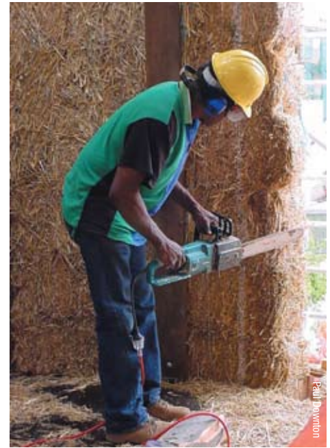
Bales are trimmed for openings and can be cut to fit structural members.
