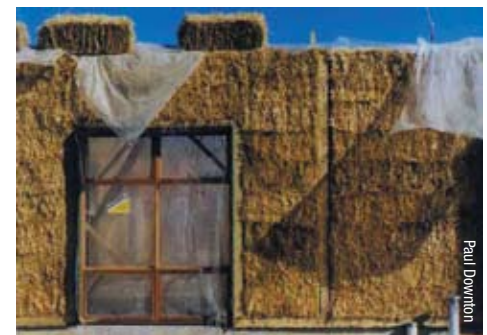
Window set towards outside face of wall.
