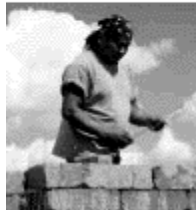
Adobe blocks were dry stacked to form the adobe walls in the demonstration house at Ganado.
