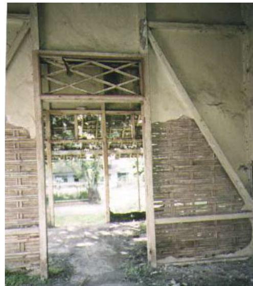
A few damaging house gave us solid proof of the bamboo mat as inner part of the wall. The skeleton could only be seen from the interior. They used mortar plaster by mixing sand with lime.
