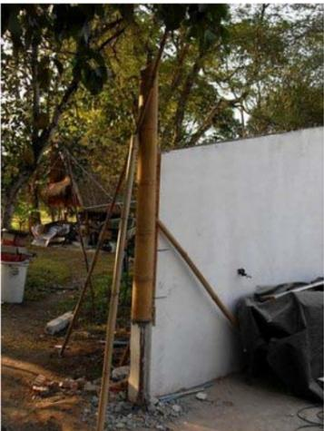
Figure 3: Bamboo Column establishment
