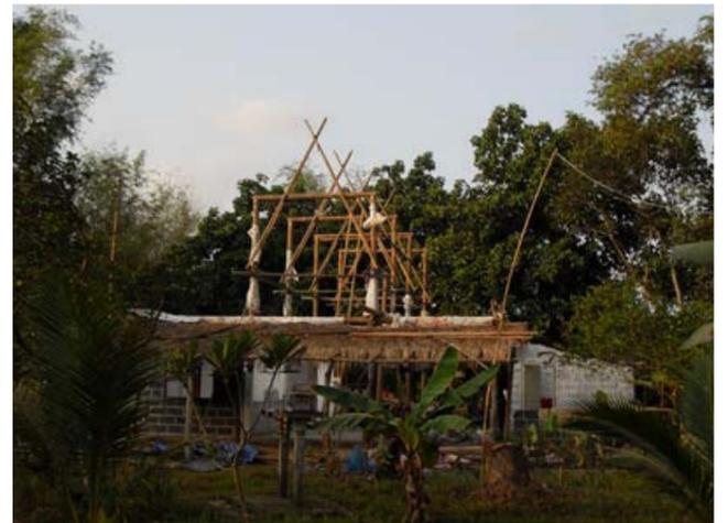
Figure 5: Triangle roof frame
