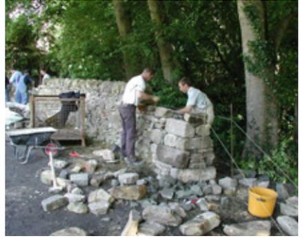
*Fig. 8 Rebuilding a section of dry stone wall – note the construction of the wall-head.*
