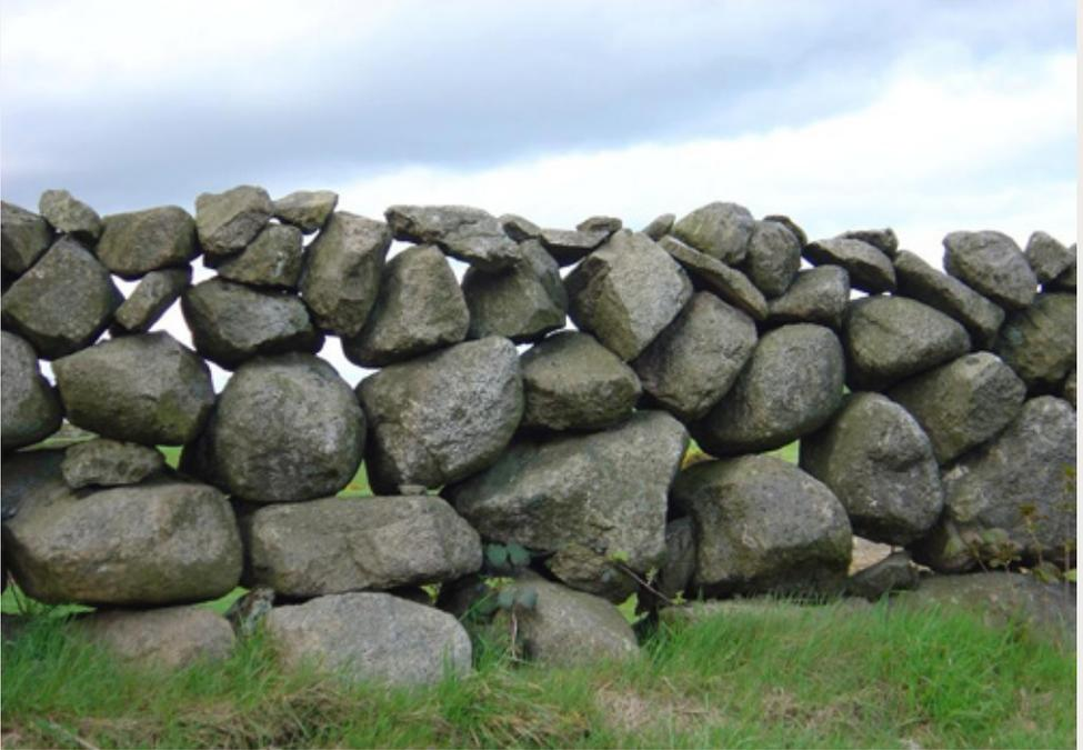
*Fig. 3 Single wall or boulder dyke.*
