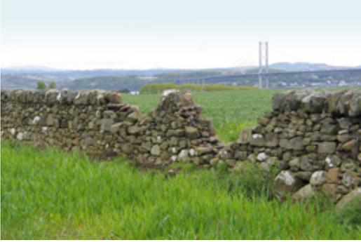
*Fig. 7 Even where a lack of maintenance has led to collapse, repair is always possible and can utilise much of the fallen material.*
