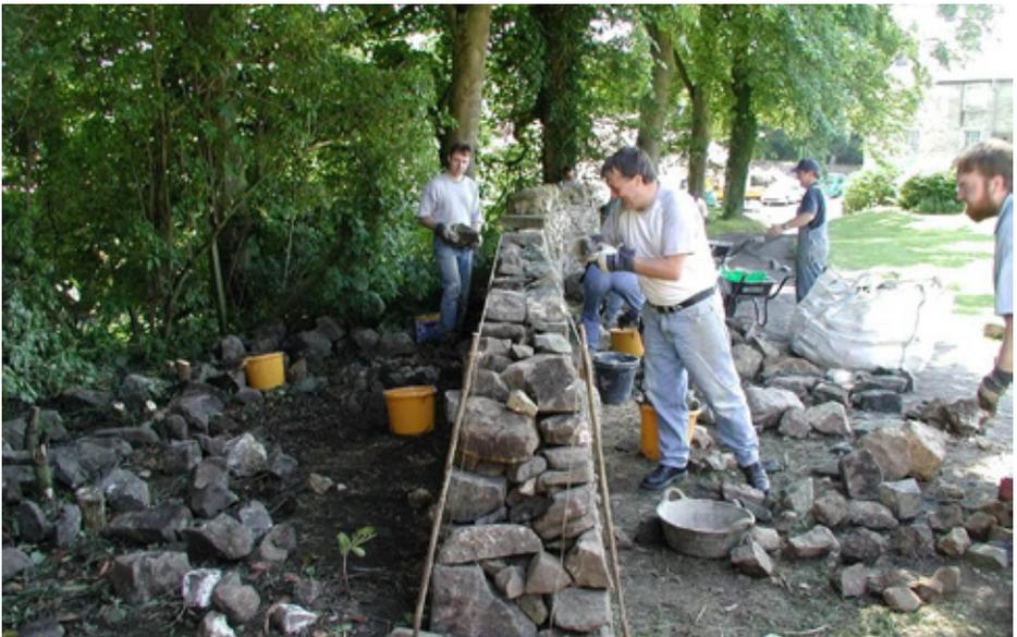
*Fig. 5 Rebuilding a section of a dry stone wall – note the use of a batter frame.*
