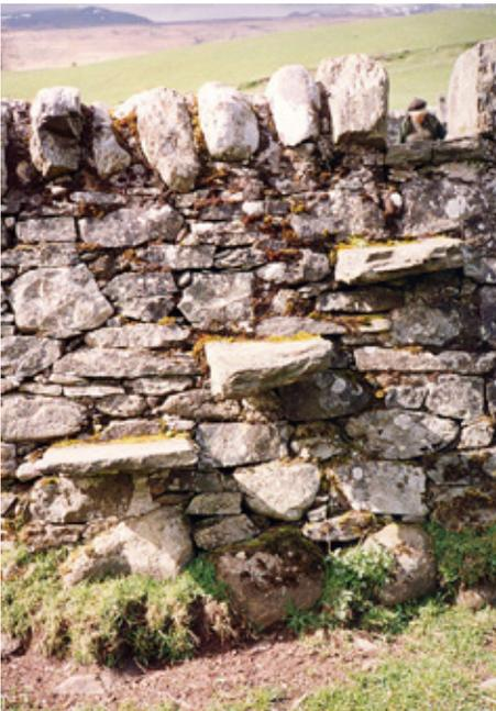
*Fig. 6 Stile built into dry stone wall.*
