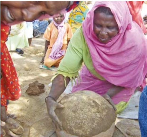
Pic 43. The mould is turned over and the clay is pressed on top of it.
