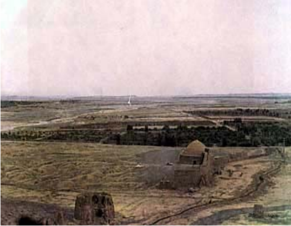
Figure 3. Earth refrigerator of Bam
